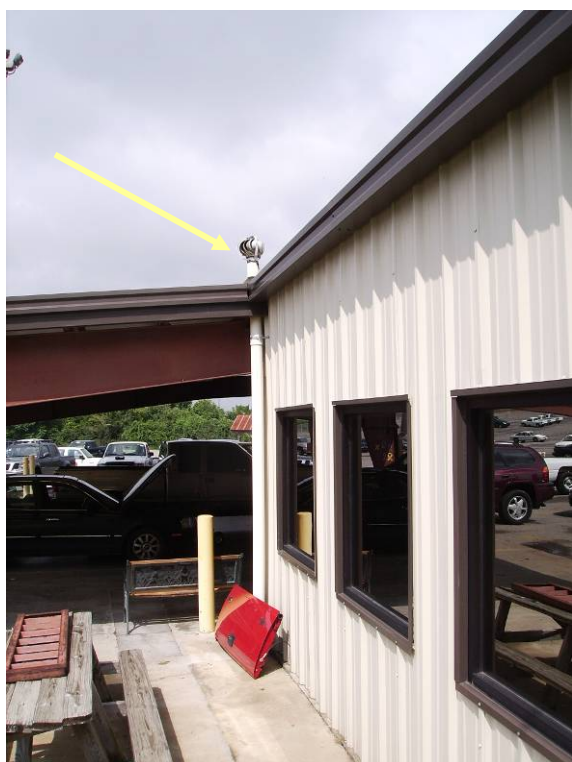
FIGURE 5. The southern side of the small graveyard building. One of two vapor vents is marked. This small building contained offices for about three employees. In the past, methane gas levels were highest within this building. A passive exhaust system was installed in December 2003 to prevent landfill gas from building up within the confined space. In December 2005, additional maintenance including caulking the floor cracks was performed to limit vapor intrusion into the building. Even with the vapor mitigation system in place, workers mentioned that unpleasant odors were often present in mornings. The building has both heating and cooling systems for indoor air climate control and ventilation.
